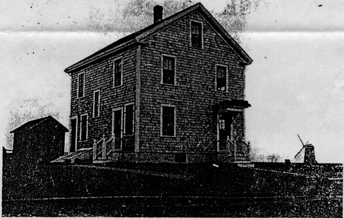
THE MELVILLE BRANCH of the Newport Post Office on East Main Road, Portsmouth is pictured in the late 1920's. Almy's windmill is in the background at right. The house still stands just north of the Citgo Station on East Main Road. The mill was near the present site of Transcom. Photo provided by James E. Garman of Portsmouth.
